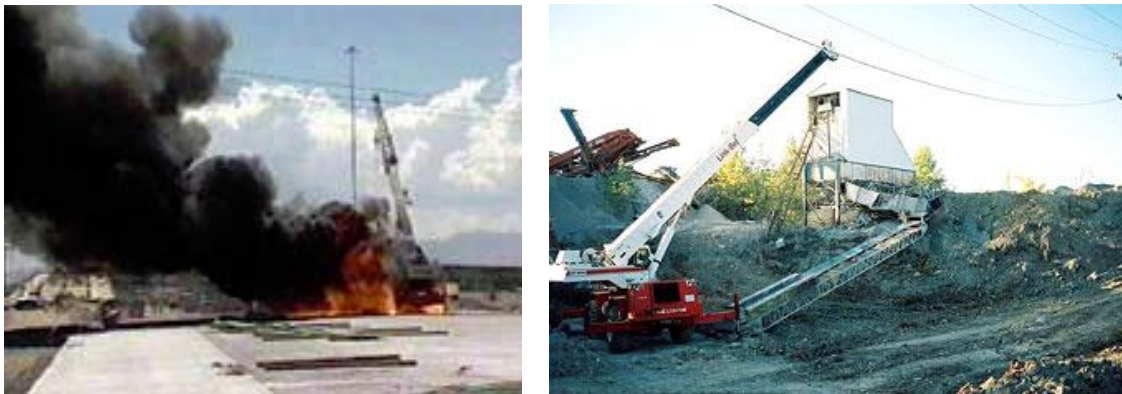
Figure 1. Fire at a construction site caused (left) and electrocution at a mine, both caused by crane contact with an overhead powerline.
